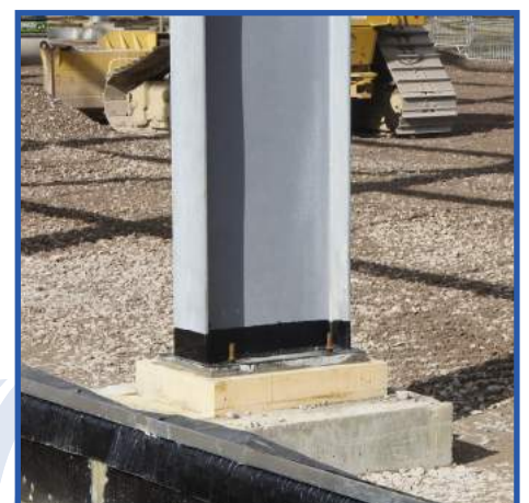
Column Base Thermal Break
